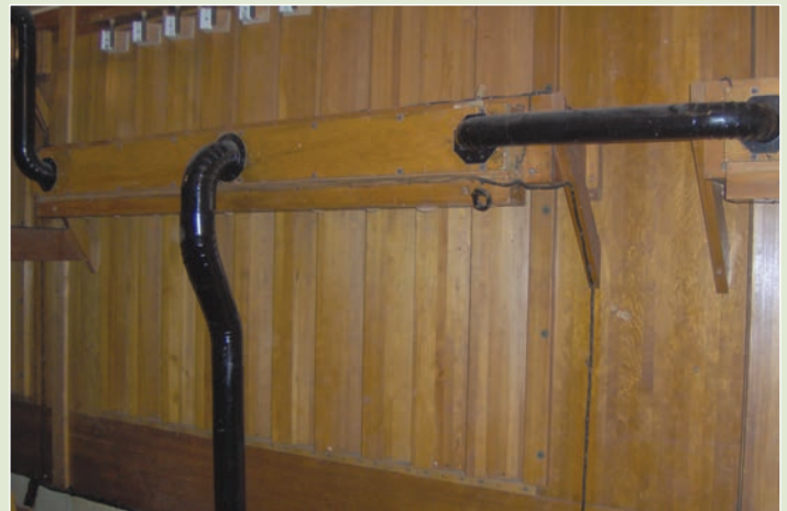
Swell shutters run wall to wall, from the height of the chest rackboards to the ceiling. The organ produces a wonderful expressive effect.
