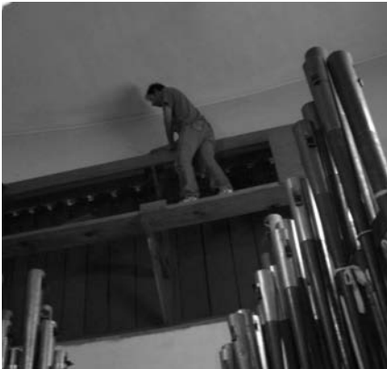
Piedmont: Chip Rainey replaces worn swell motors 25 feet up (Photo by Buddy Boyd)
