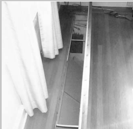
Opening in living room floor—mixing chamber below
