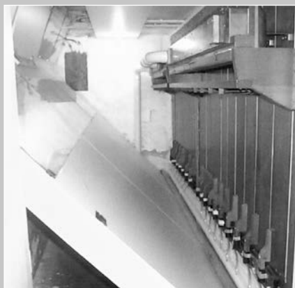
Mixing Chamber: Shutter frames installed with actions on the exterior.
