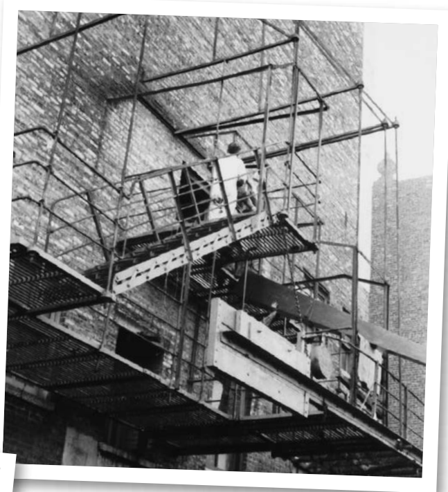
A 16' Diaphone resonator exits through the fire escape
