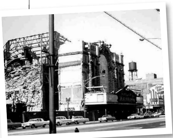
The Marbro is demolished, 1964
