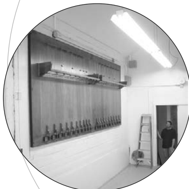
Solo chamber following installation of the swell shutters from Opus 2155 (Photo by Carlton Smith)
