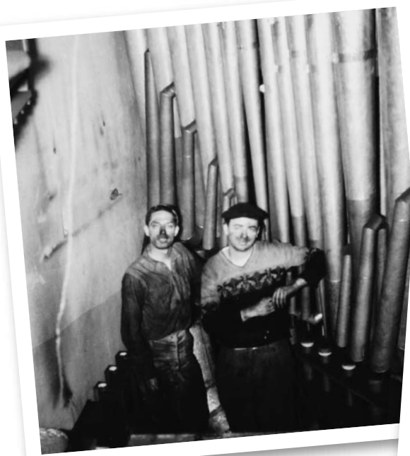
Bob Richards(L) and Jon Habermaas with 16' Tuba pipes
