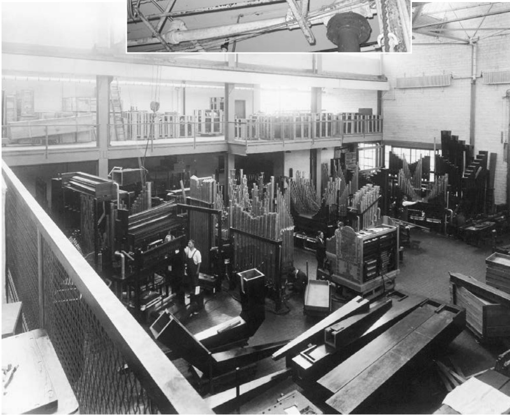
The same mezzanine and railing are seen here eight decades ago, in happier days. The organ being tested is Opus 1953 destined for the Fisher Theatre, Detroit
