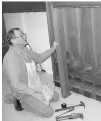
Inland Empire: Stuart Goodwin installs a bass chest for the Style 150 Wurlitzer (Photo by Jim Henry)
