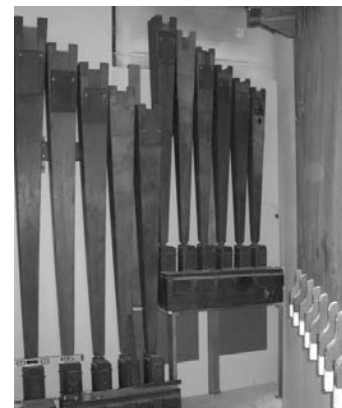
Eastern Massachusetts: Diaphones in Main chamber of Hanover Theatre (Photo by Bruce Hager)
