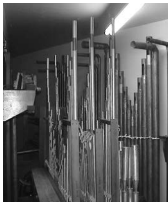
Puget Sound: Repaired plaster and re-installed pipes (Photo by Tom Blackwell)
