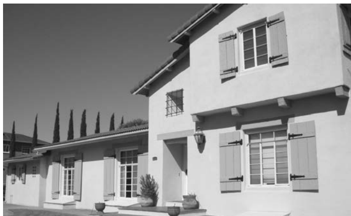
Exterior of residence (Photo by Ray Carnovale)
