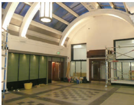
Purpose-built organ chambers with high-level tone openings and glazed viewing panels below; the console will be garaged between the chambers
