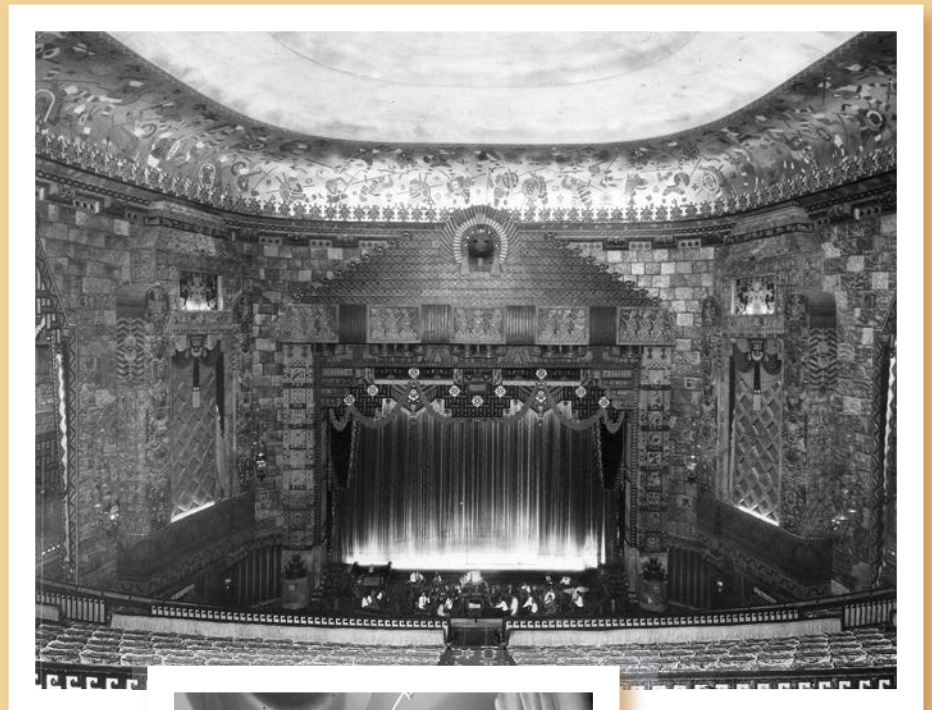
Site of Wurlitzer Opus 1953's original installation, at the Fisher Theatre, Detroit
