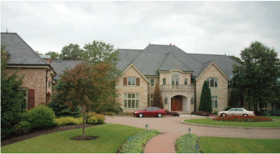
Exterior of the Aveni/Villarreal residence
