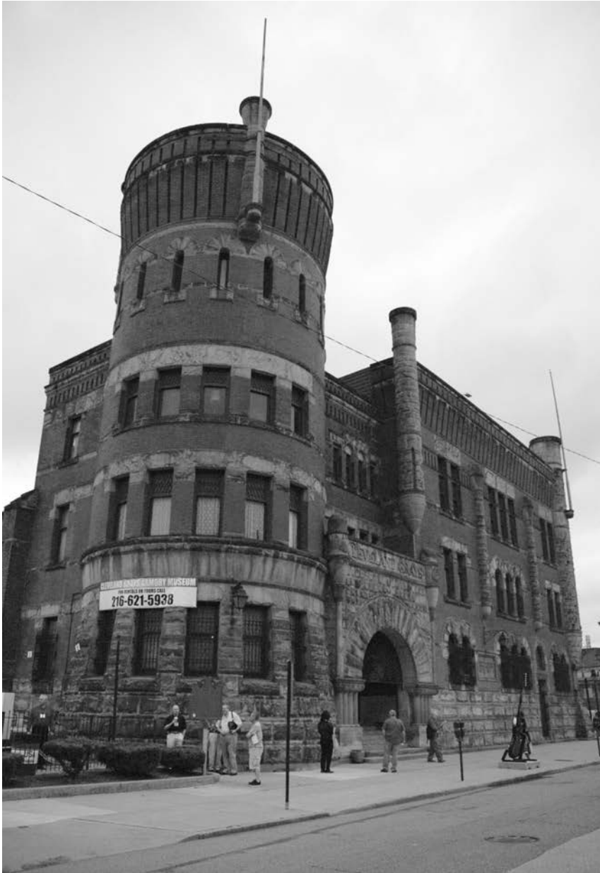
Exterior of the Cleveland Grays Armory (Photo by Richard Neidich)
