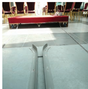
The guide track to ensure perfect location of the console when garaged
