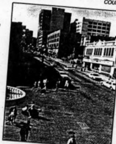
Top - The silhouette of the Liberty Theatre's monumental sign (trolley) holds its torch above a crowded street scene on First Avenue near the Pike Place Market. Above - A parking lot replaces the theater, long a landmark in the downtown area.
