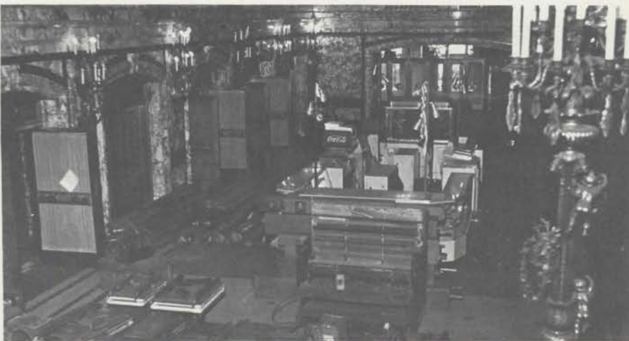
The lobby of the Paramount serves as the final departure point for parts of the Mighty Wurlitzer. Square items in foreground are bellows for the instrument. To the left of the snack stand are some of the many ranks of pipes. The piano mechanism is immediately in front of the snack bar.
