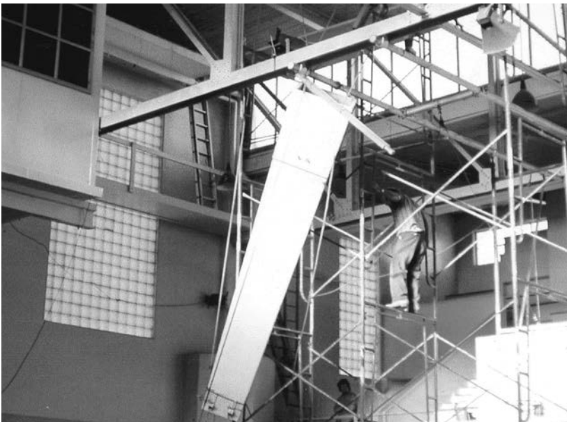
The Diaphone is lowered in sections (SFNTOS archive)
