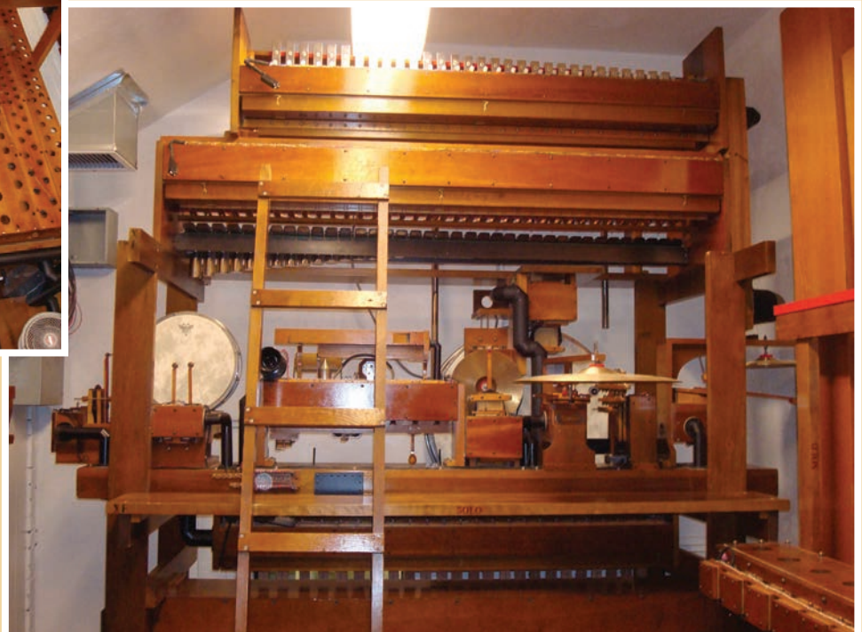
Solo percussion tower during installation
