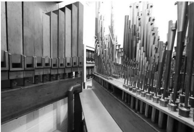
Rear of the Solo chamber. Notice the workmanship on the PVC wind line on the Tibia offset (Lance Luce Collection)
