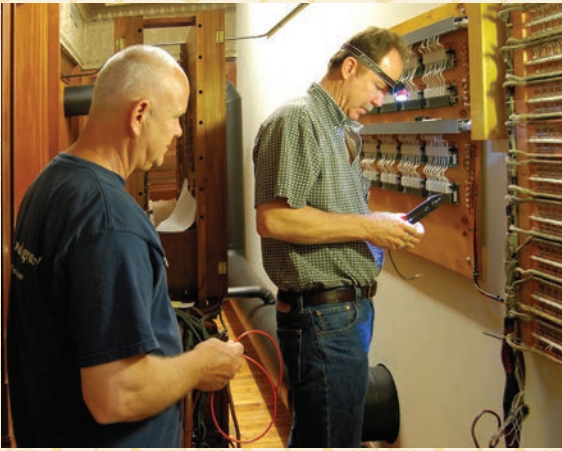
Roger Lane and Bob Knight work on the player in the relay room (Everett Sahrbeck)
