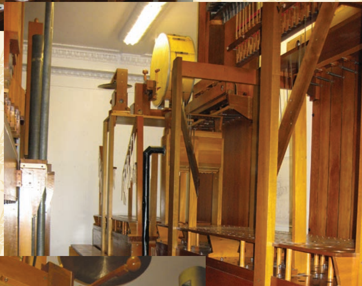
A view from the chamber door of the completely assembled chests just prior to fabrication of new windlines (Jim Stemke)
