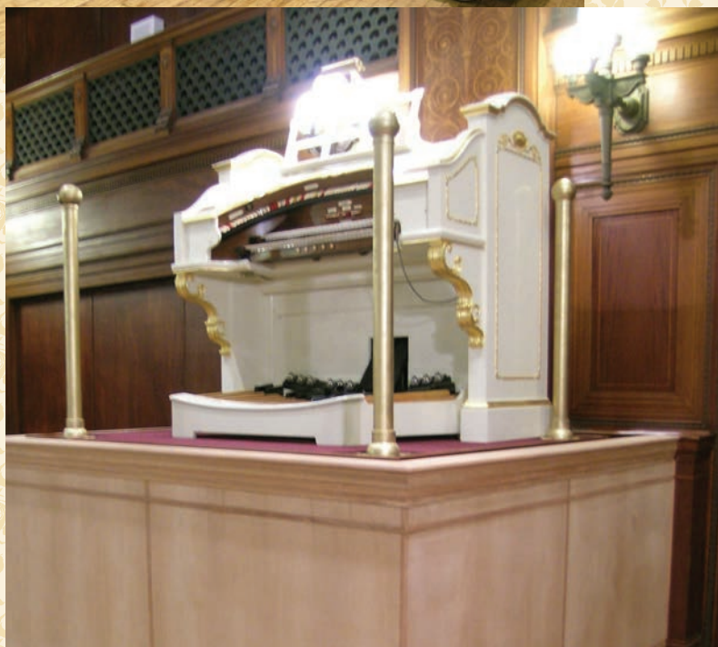
The decorative wall around the console and lift prior to finishing. The wall was handmade by shop woodworker Scott Kip (Scott Kip)
