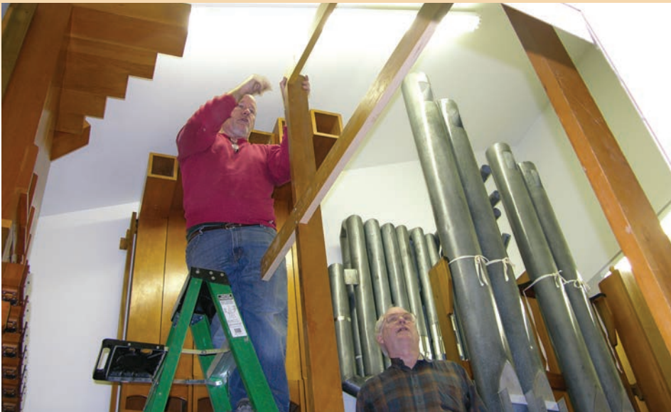
Bob MacNeur and Rob Kingdom installing part of the racking for the percussions and traps. They will mount above the manual chests. The 16' Salicional and 8' Diaphonic Diapason are visible behind Rob (Photo by Mike Bryant)
