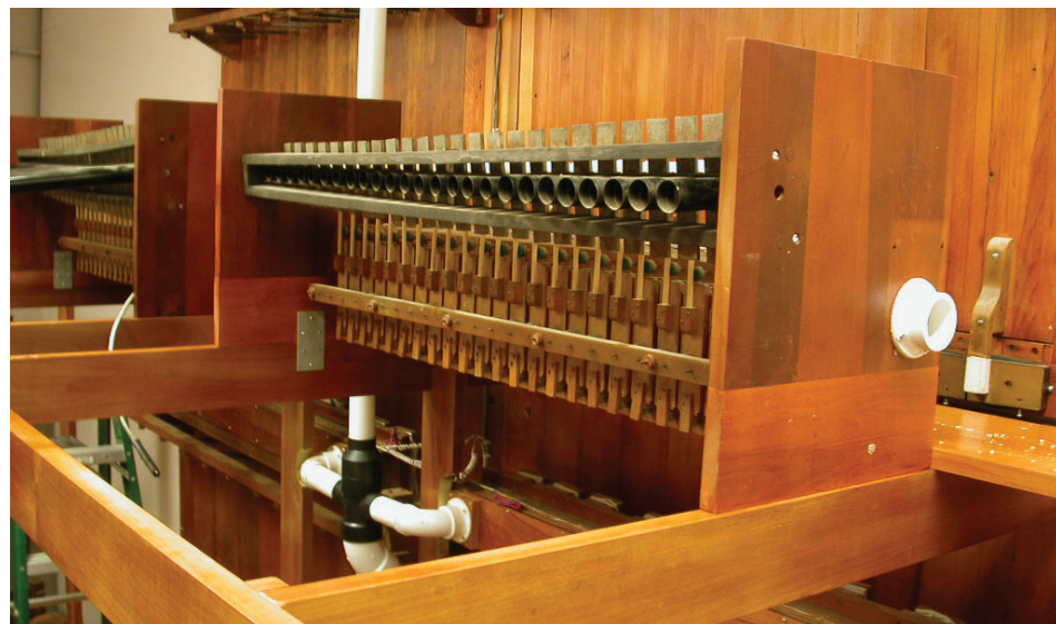
Chrysoglott installed, Main chamber
