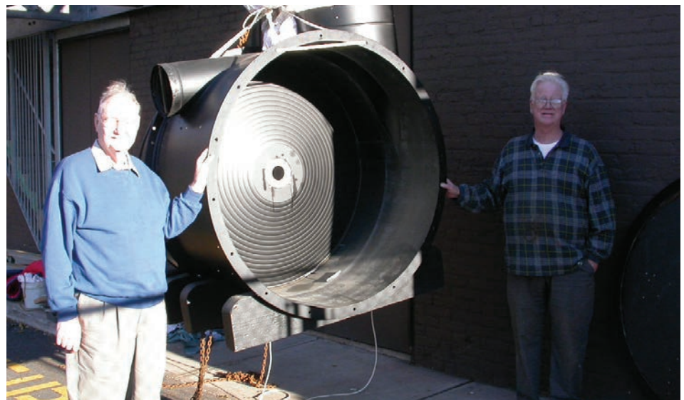
Ken Duffie (L) and Don Phipps prepare to send the blower aloft
