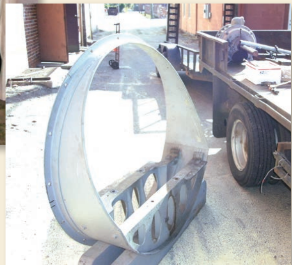
The blower tank had to be disassembled as much as possible to make the turns in the stairwell going to the blower room
