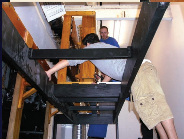
Wilson Luna and Patrick Hodges (of A.E. Schlueter) installing percussions
