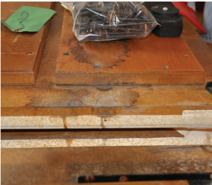
Water-damaged regulator (Photo by Matt Madden)
