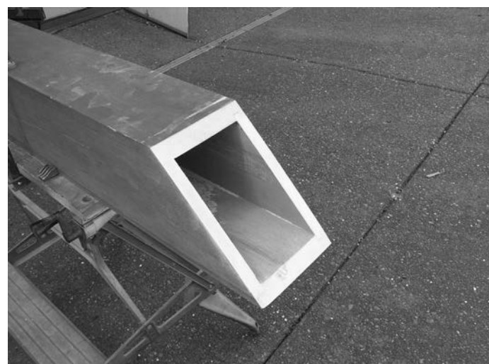
Figure 10. We're ready to mark and drill
