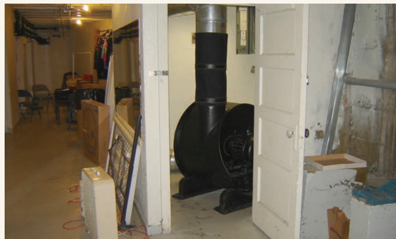
The restored blower installed
