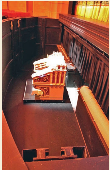
Console in the pit; the console is stored beneath the stage, and rolled onto the lift when needed
