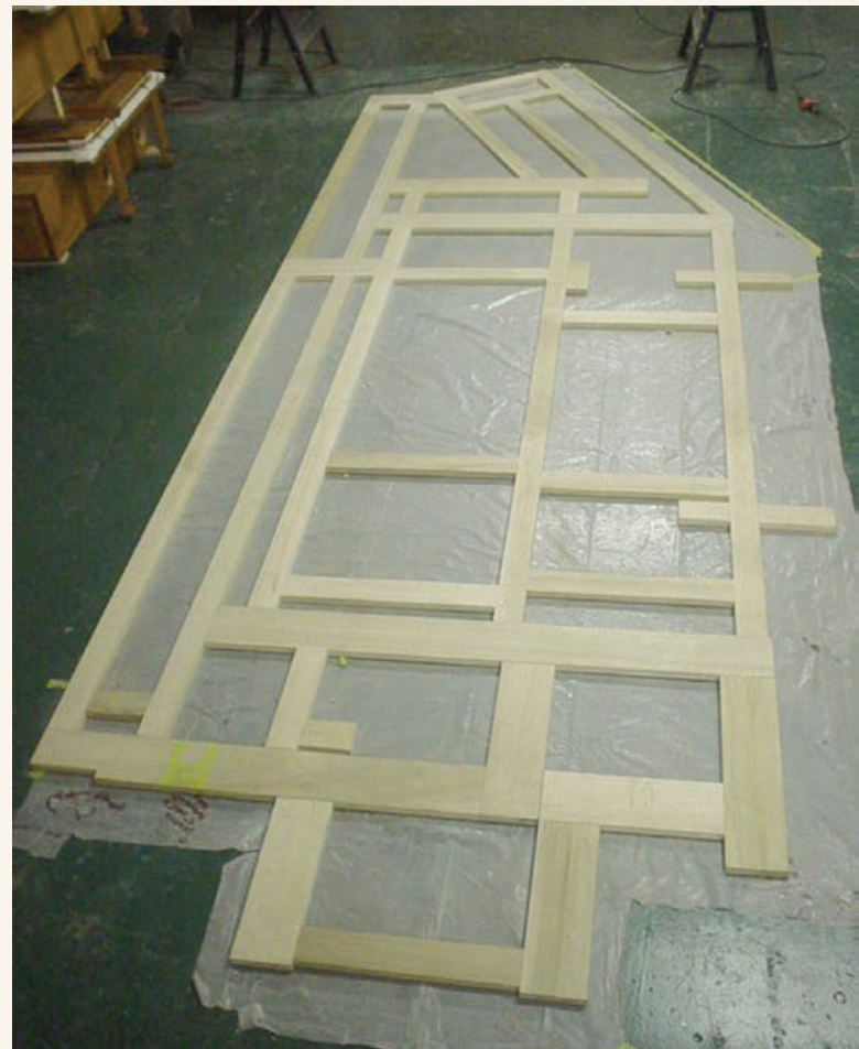
A new ground frame for each chamber was made; this is the Solo frame
