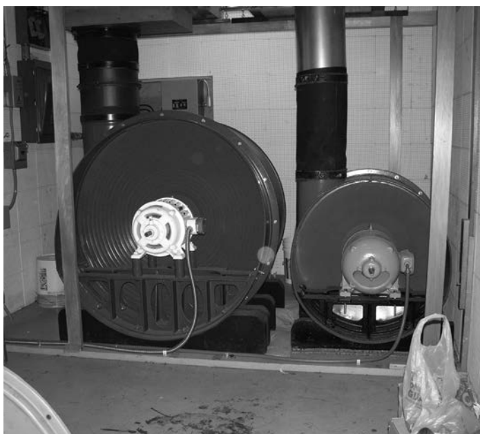
The large blower on the left is for the low-pressure organ; the smaller blower supplies the high-pressure side
