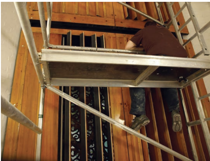
Solo shutter installation
