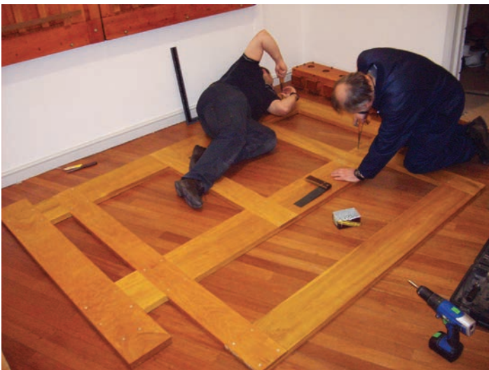
Installing lower Main ground frame
