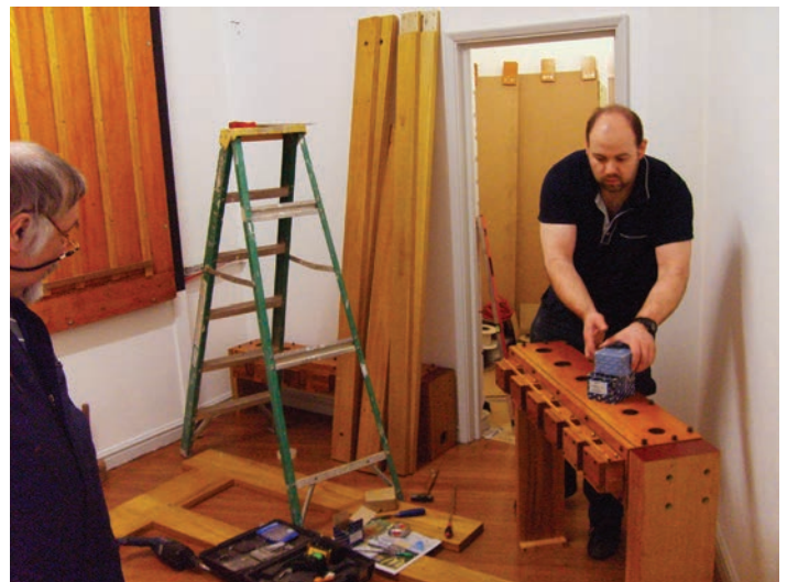
Lower Main installation
