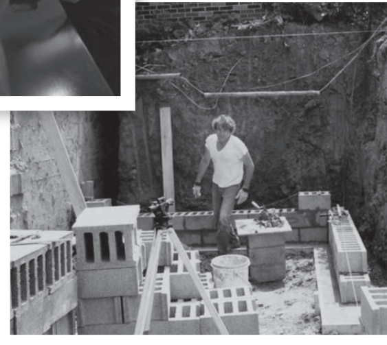
Don laying cement blocks for Music Room (Photo by Ben Robertson)
