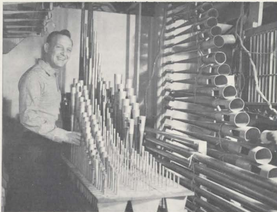
When Tubas and Strings are too high for the ceiling, install them horizontally! View in Main Chamber.
