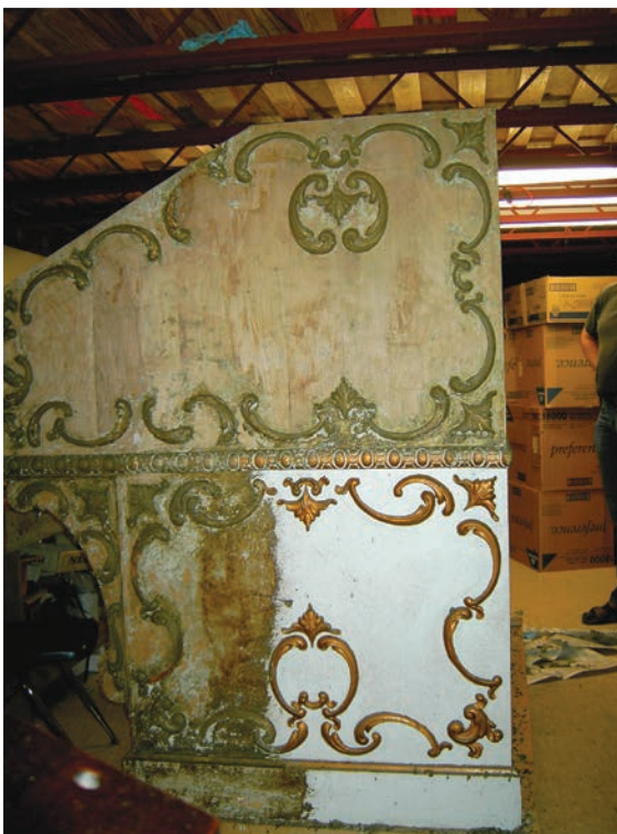
In 2003 the old finish was carefully stripped, leaving the decorative moulding intact
