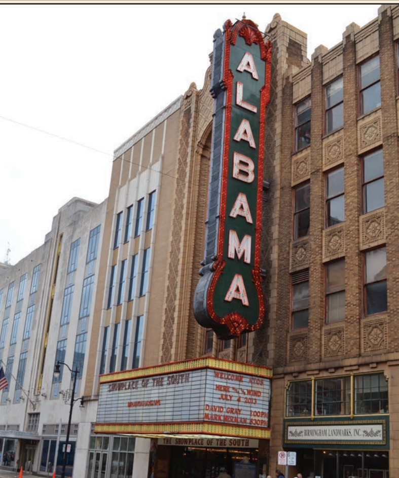
Across the street, the Alabama Theatre ("Showplace of the South") welcomed us (JS)
