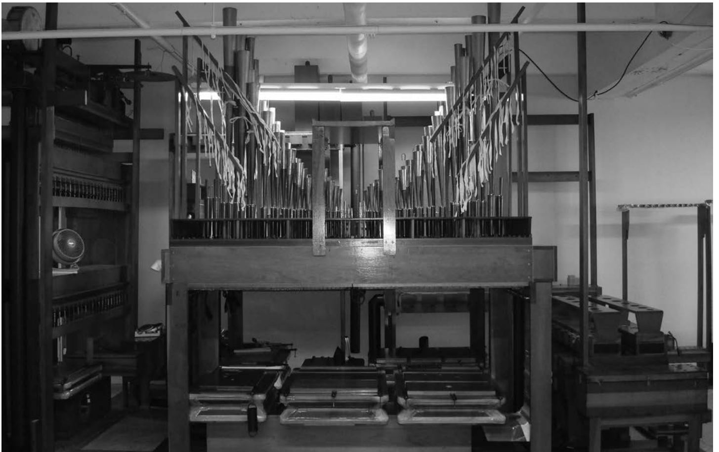
Before the organ was moved into the chambers, it was erected in Carlton Smith's shop. Here's the Solo chamber in the erecting space: note the percussion stack on the left
