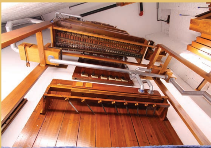
The Solo chamber, mid-installation, with winding complete, before pipes are installed
