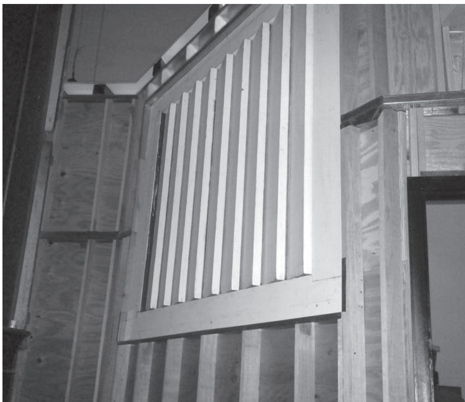
Solo chamber under construction
