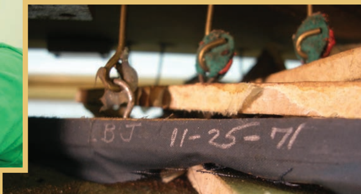
Each pneumatic Len Johnson recovered was dated and initialed, such as this switch board secondary, recovered in Polyton. Original zephyr covering is visible on other pneumatics
