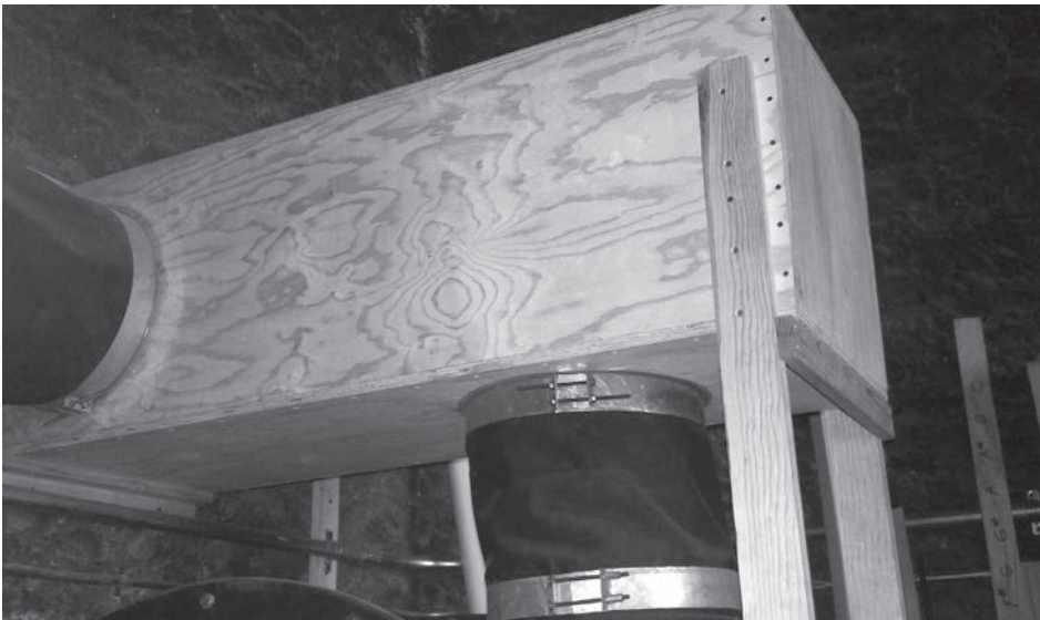
A muffer box helps to reduce wind noise through the system
