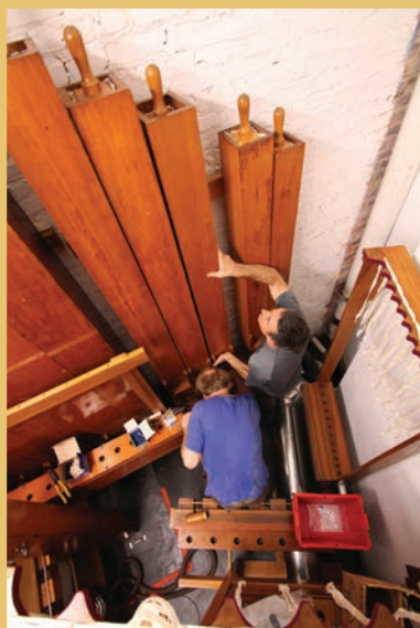
Erik Spooner and Joseph Rotella install pipes of the 16' Bourdon in the Main Chamber
