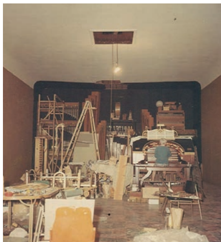
Installing the organ in the theatre (Bill Field Collection)
