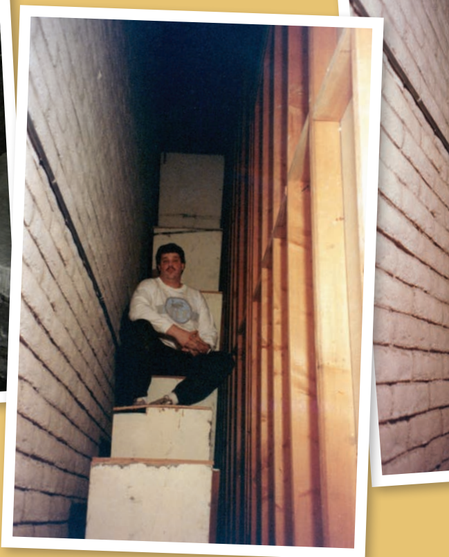
The 32' diaphones in 1992 had a stairway built above, following the length of the resonators (Photo by James R. Stettner)
