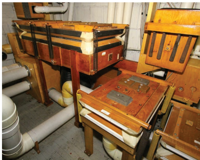
Three of the nine regulators in Main chamber (Photo by Lance Luce)
