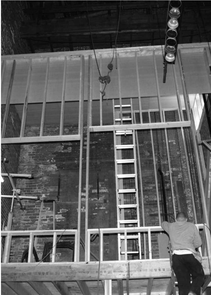
Construction of the rear Solo chamber in the Colonial Theatre
