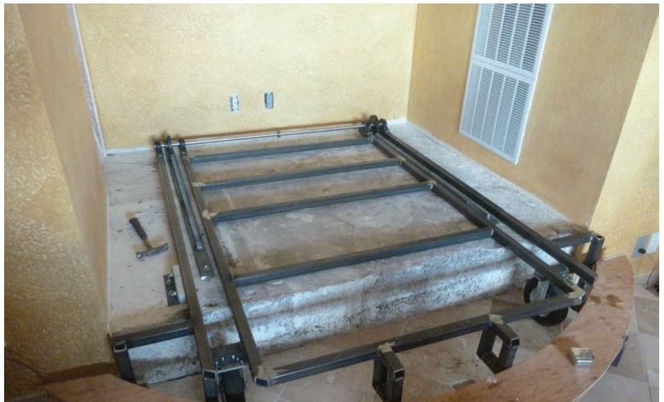
The steel frame for the console platform
