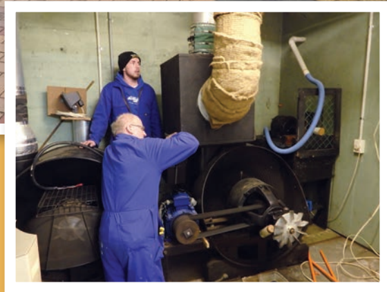
Steve Crawford and son James begin dismantling the blower plant (Photo by Laurie Mathews)
