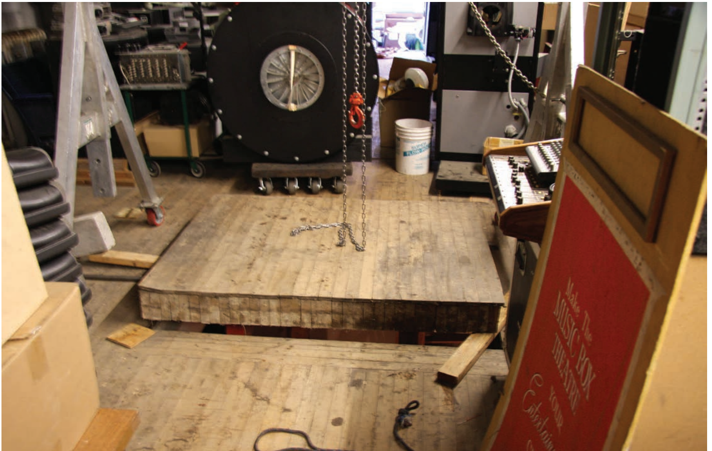
The riggers have set up the rigging and are removing the trap from the floor; the blower is on a dolly, ready to go
