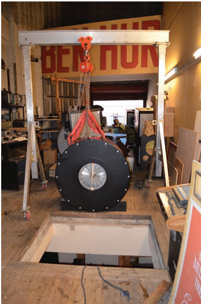
The blower is strapped in, ready for the lift
