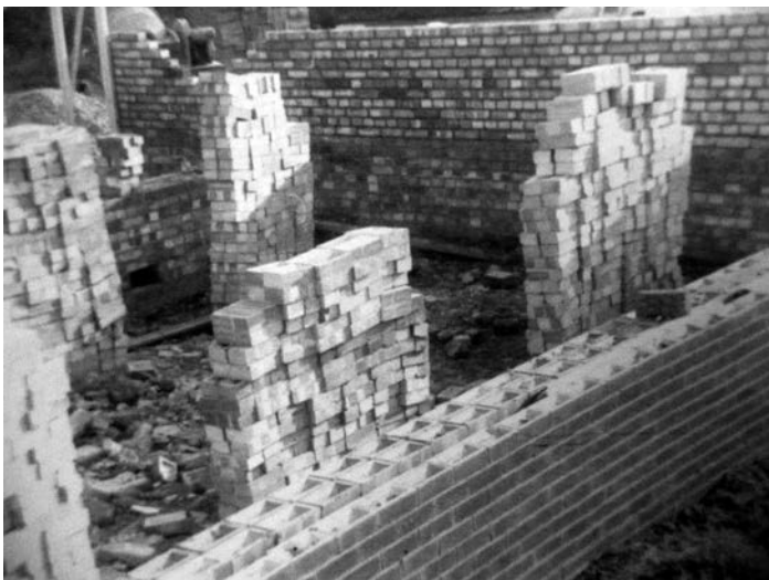
Organ chamber construction at Chorleywood (Len Rawle collection)
