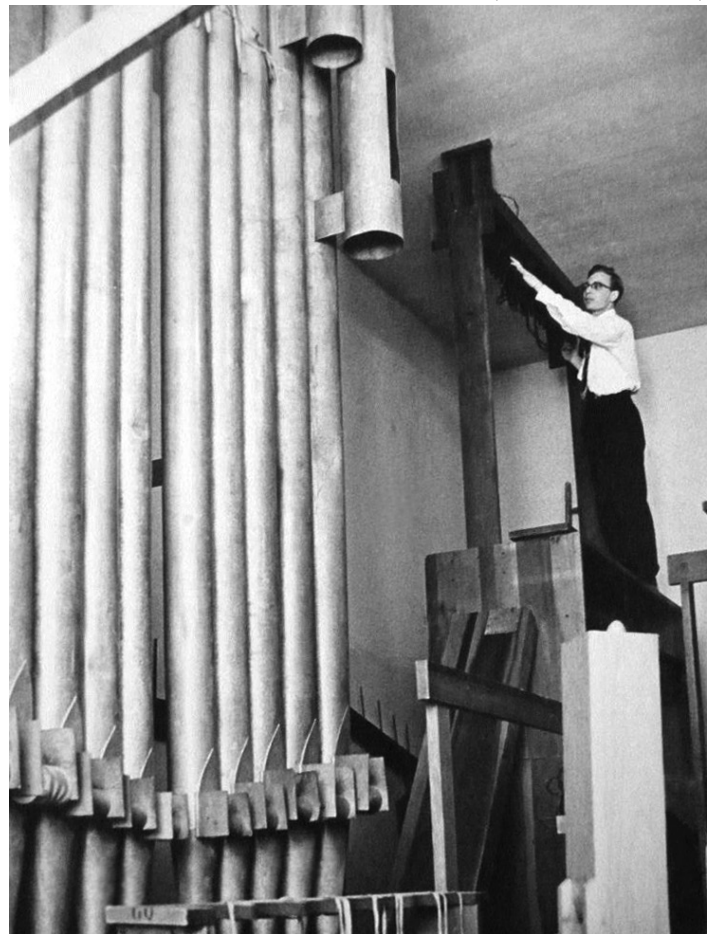
Main division installation—16' Gambas (Len Rawle collection)
