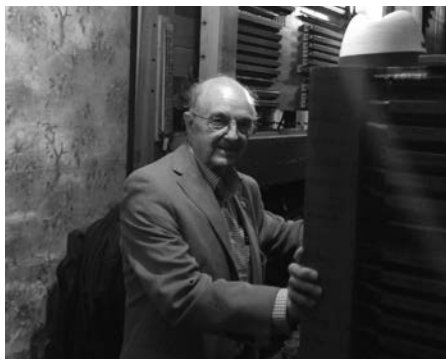
Edward M. Stout III in the relay room of the Castro Theatre. In well over 30 years of heavy use the original Wurlitzer relay required only nine minor repairs (Photo by Roy Powlan)
