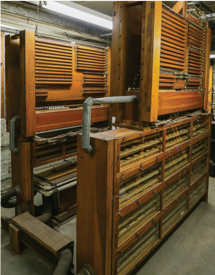
Armory Relay Room (Photo by Geoffrey Powers)
