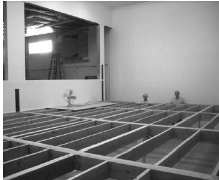
View from inside chambers with doubled 2x8s marking chest bearing positions and the divide between chambers. Yes, that would be Dick and Ed at the back.
