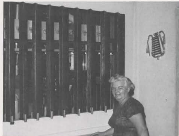
Ruby Derby stands before one of the two sets of swell shutters which control the organ's volume. Chambers are each 12' x 12', 20' high.
