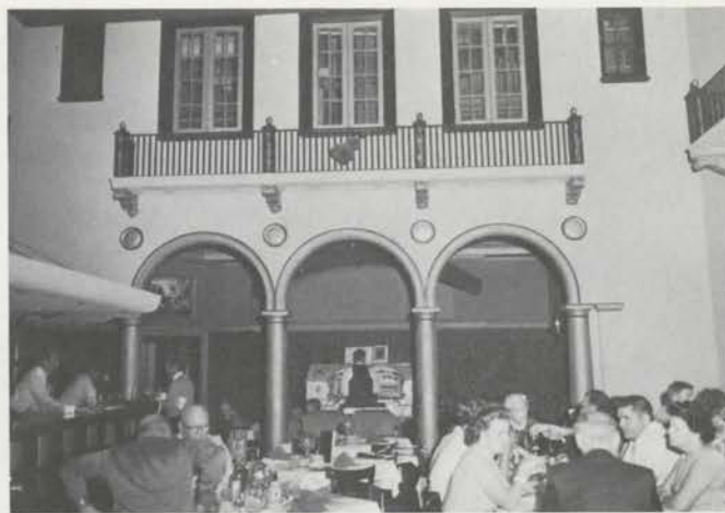
The Colonnade Room. The Mansion is U-shaped and this was the open courtyard before being roofed over. Note the pipe-work behind the balcony windows and the console beneath the center arch. The restaurant also boasts an Estey horseshoe electronic organ and a square piano.
