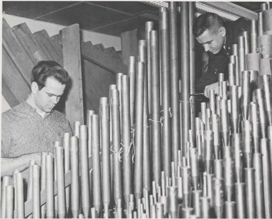
Potomac Valley Chapter members Bob Oberlander and Paul White are hard at work on the installation of a Moller 2-10 in the studios of advertising executive and local WPIK broadcaster Doug Bailey. Pipes for the organ are from the 3-31 Moller formerly in the Loews Palace Theatre, Washington, D. C., and the console controlled, at one time, the organ in the old Shoreham Hotel, Washington. The organ is used every day for broadcasting on the afternoon Doug Bailey Show, and also over a local FM station in nearby Bethesda, Md. Both Oberlander and White have sizeable residence installations in progress, and Oberlander is currently installing a 2-6 Wurlitzer in the Baronet Theatre in Bethesda. The Baronet, formerly the Hiser, had a 2-5 Marr & Colton which is now in the residence of member Wendel Hill.
