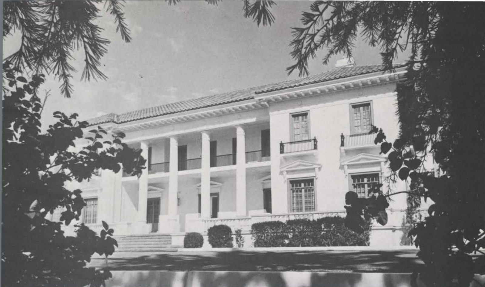
The River Mansion restored to its remembered elegance.
