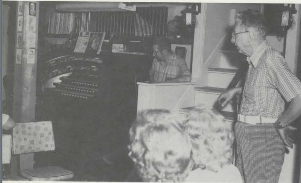
Dave Brewer (center) and his father (right) are proud of the Marr and Bartolitzer installed in the basement of their home.
