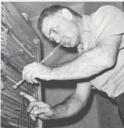
ROSS FARMER brushes dust from switch stacks. Organ unification switches are among the hardest, most dependable types known, but must be used often to prevent oxidation.
