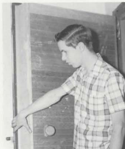
KEN KUKUK examines the 8-inch-thick refrigerator doors which seal in sound. The original specification called for these sound barriers at entrances of all chamber and blower rooms.
