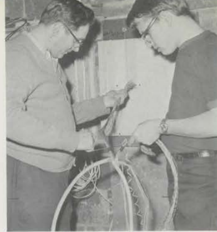
Marvin Lautzenheiser (left) and Paul White at work on part of the console cable.
