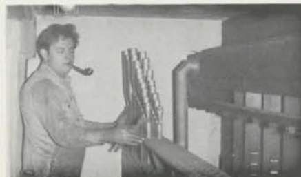
Neal Kissel removes the last of the Vox pipes from their chest in the Albee theatre to pack them for the long journey to a new home in California. Neal is in charge of the detail readying the 3-15 Wurlitzer for installation in the San Gabriel civic auditorium.
