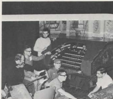
Console in place.
