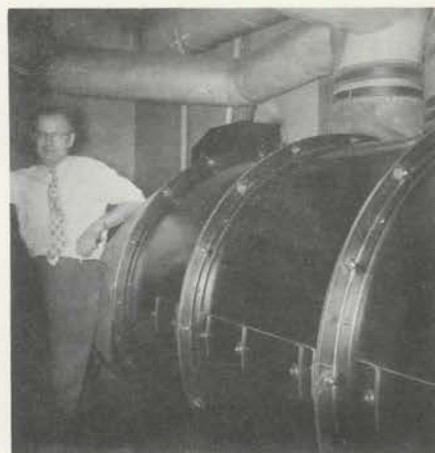
Dan Papp inspects the New York Paramount's mighty wind supply (1957).
