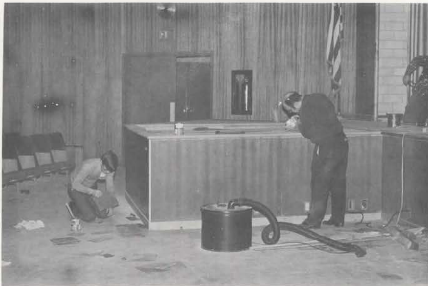
Dave Mudruch and Bob Dilworth working on organ pit.
