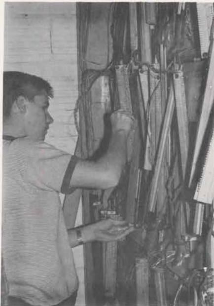
Bob Wilhelm wiring the switch stack.
