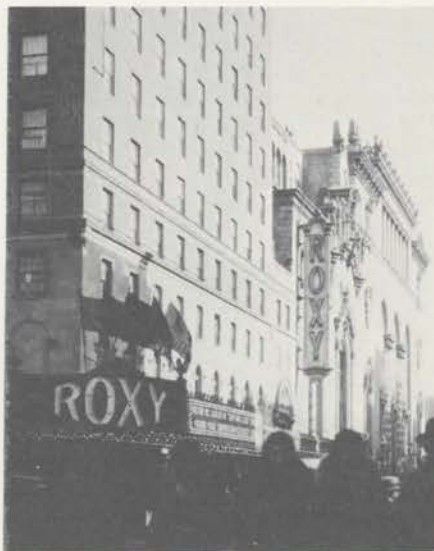
The full magnificence of the structure became apparent only after one left 7th Avenue and walked down the one-way side street, as shown in these 1927 photos shot by Clealan Blakely. (Opposite page also.)
