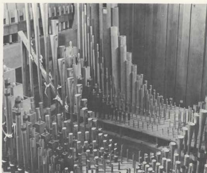
MAIN CHAMBER AS IT WAS. Firemen chopped a hole in the roof and poured water and chemicals into the chamber. What the fire started, liquids finished. No useful pipe or chests remained. (1964 photo by John Craig)
