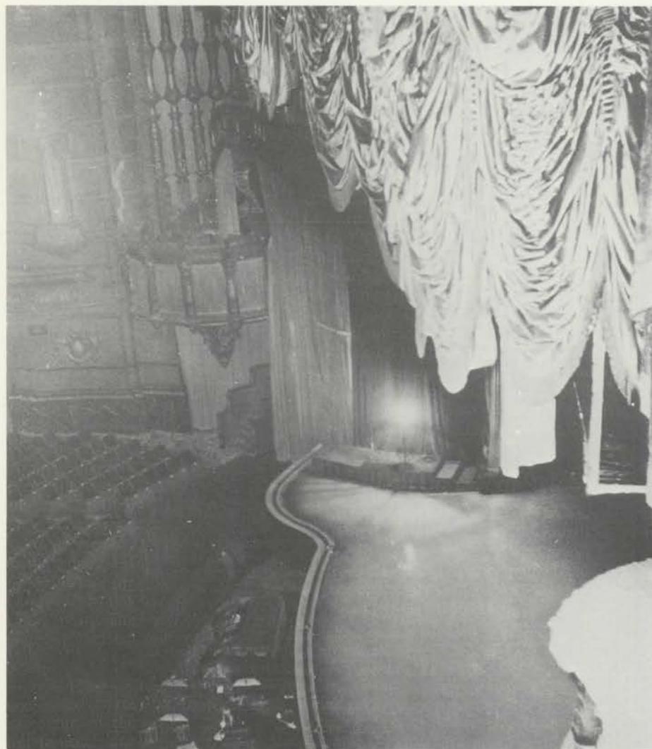
The 'Ice Age'. This photo shows how much the stage was extended to nearly obliterate the once huge orchestra pit. It is seen here after it was flooded to provide an ice surface for shows presented on skates. When this photo was taken (in the '50s), the console could be seen in the pit. It spent much of the 'Ice Age' perched on the little balcony (left of center).
