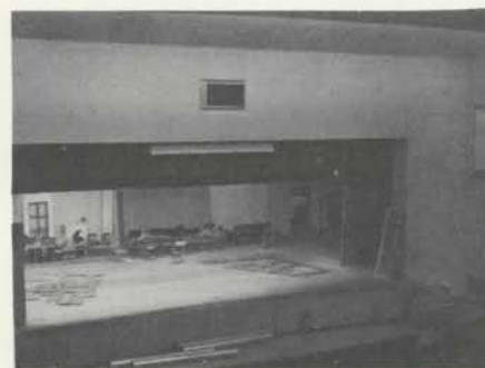
Chamber floorboards laid out on stage before installation in chambers.
