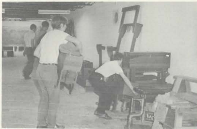
Converted indoor rifle range offers large well lighted and clean area for renovating the Wurlitzer. Here the first parts are being placed in the room which is over 100' long.
