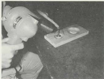
Using a heat gun to form pouches. Simple device is used to achieve uniform depth of pouches.
