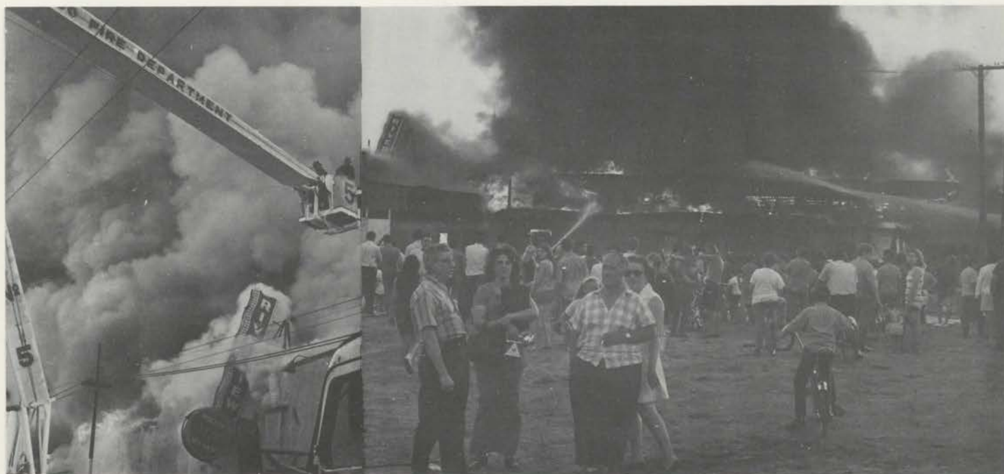
Wall and sign have collapsed. Intense heat blistered the paint on the Chicago Fire Department snorkel.
