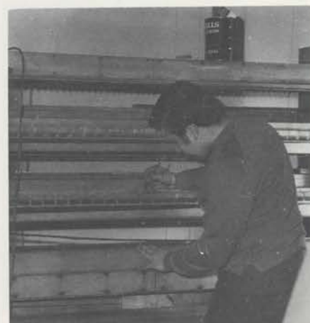
Art Todesco adjusts contacts on relay.
