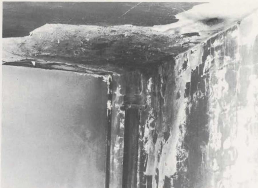
Damage to ceiling and wall of right chamber caused by years of water seepage from a leaky roof. Luckily, no irreparable damage resulted.
