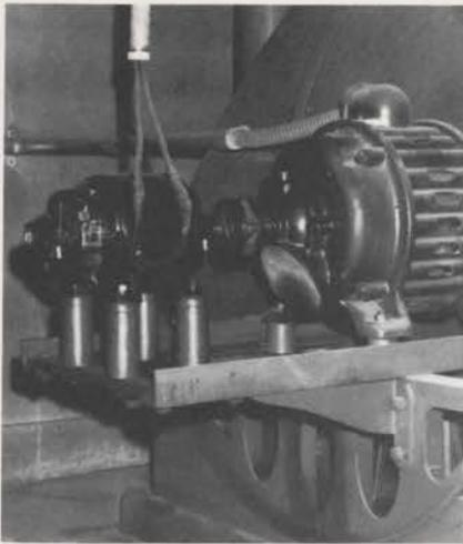
The 15 volt, 22 ampere generator runs from the driveshaft of 15 hp 440 volt 3 phase Woods motor. The Orgoblo (right) generates 10 and 15 inch pressures. Blower room is off the right chamber.
