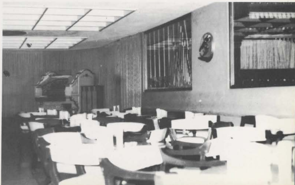
General view of the Panama installation. The overhead grille is the tone chute. Pipework can be seen through windows.
