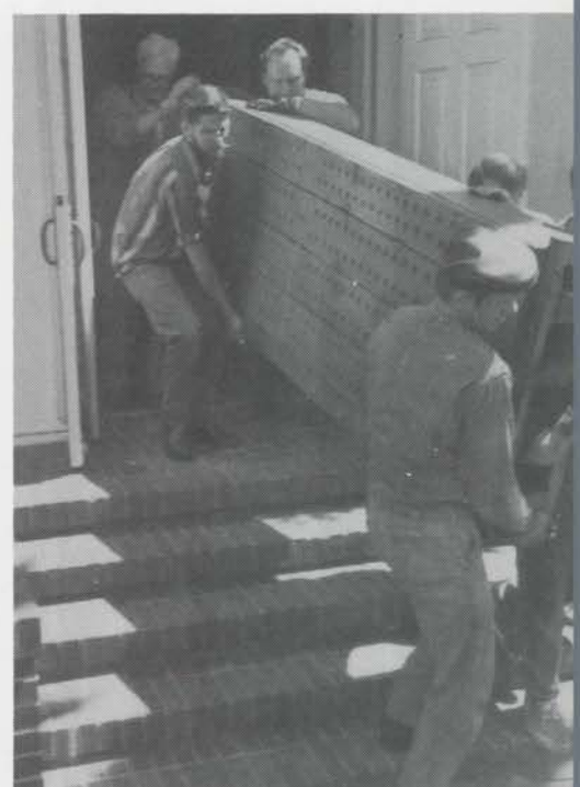
Too large for the side door, the chest takes the same route as the console, up the center aisle and out the front door.
