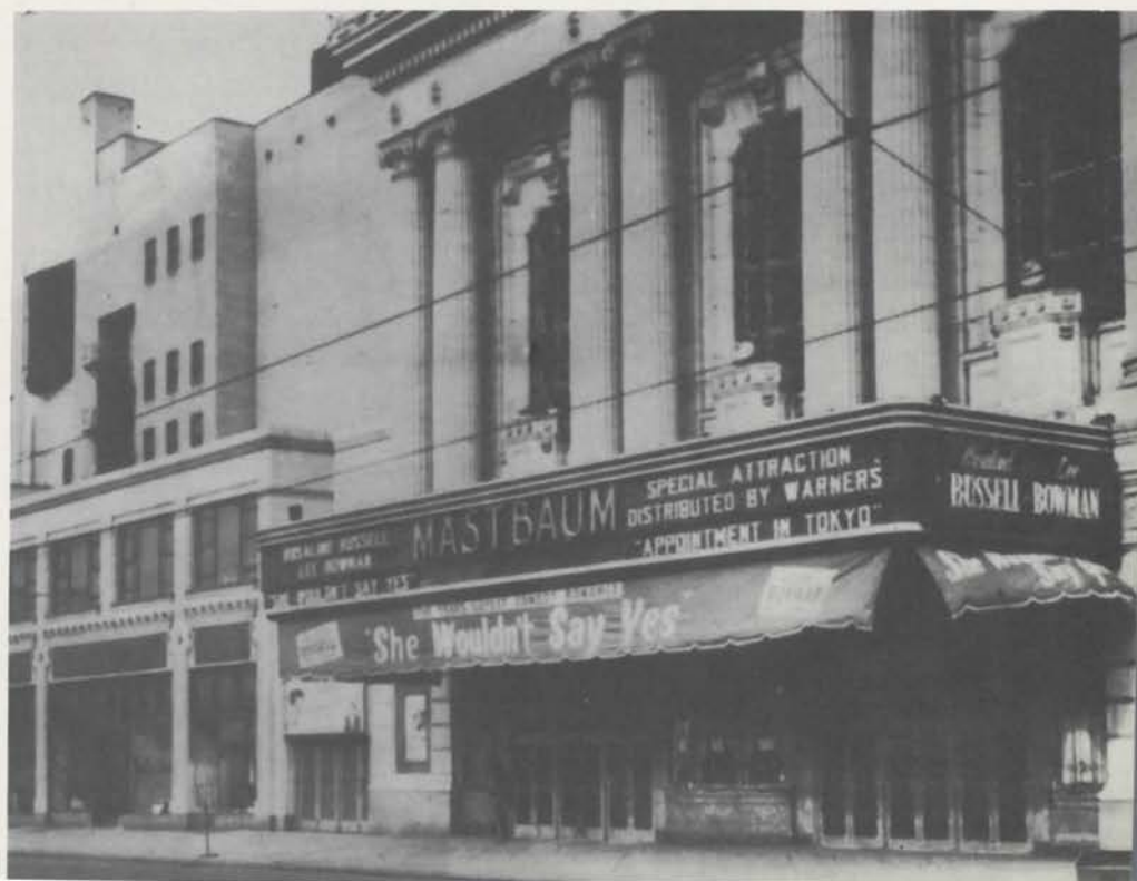
The 5,000-seat Mastbaum Theatre about December 1945. Often beset with labor troubles during its history, it was the most beautiful theatre erected in Philadelphia. — (Philadelphia Public Library)
