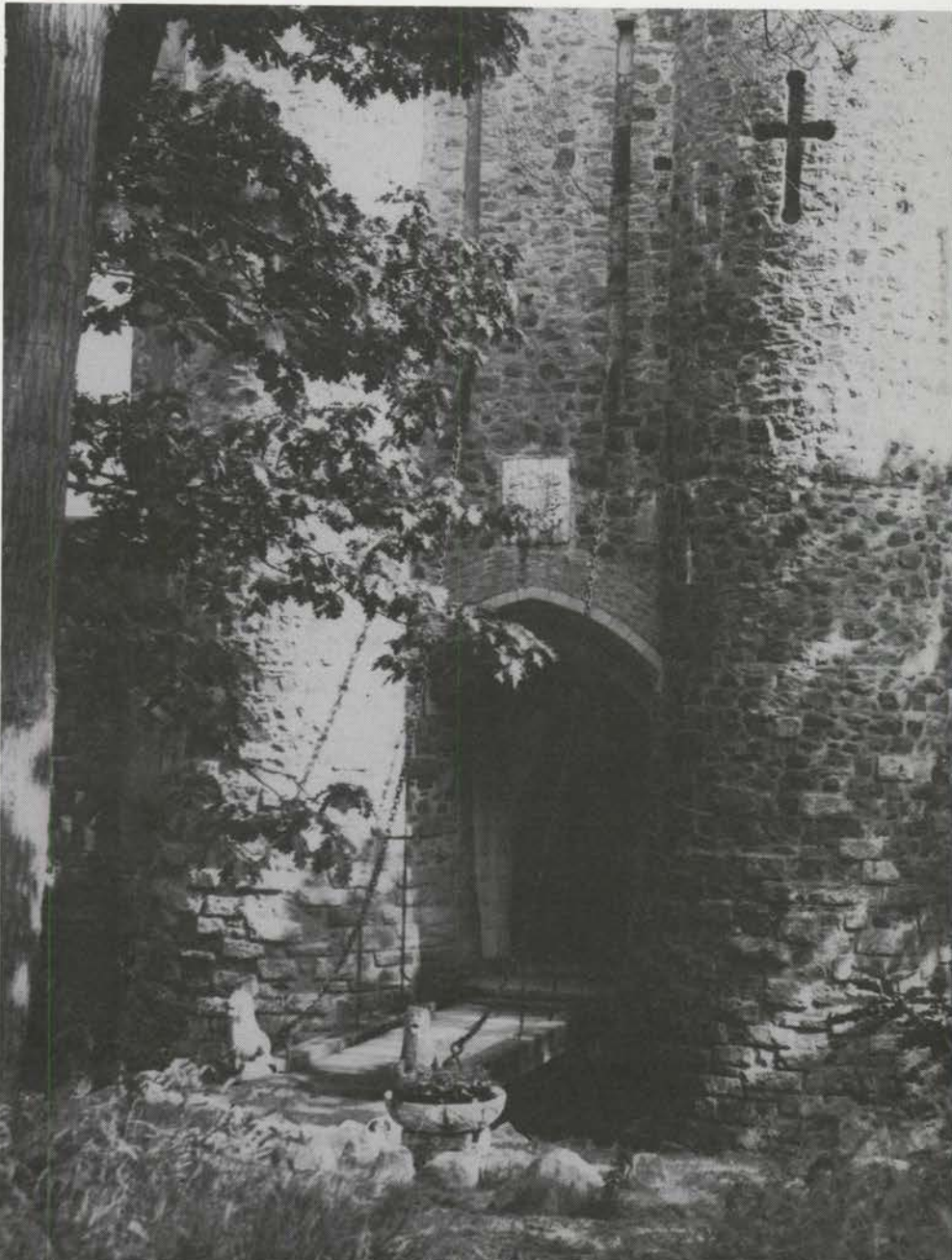
The Hammond Museum . . . a 1928 version of a medieval castle, complete with drawbridge and moat.
