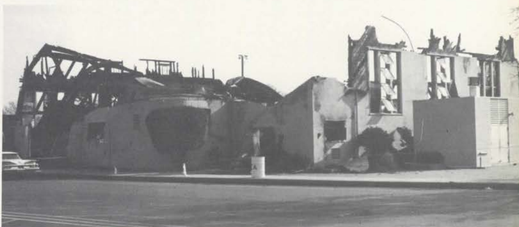
All that remains of the boys' gymnasium. The main school building and auditorium is west of this location. Note the window panes. These are a plastic material which is becoming popular for use in locations where windows are subject to frequent breakage. — (A Carroll F. Harris/Harold Baxter Photo)
