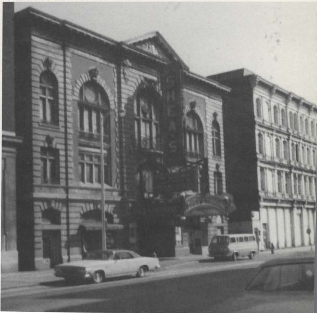
Shea's Theatre, Erie, before demolition in 1968.
